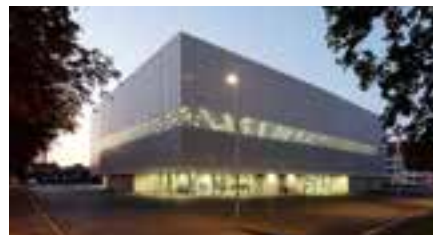
Sporthalle Hardau, Zürich - Garderoben
